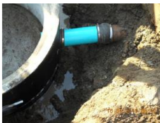
Typical modern rubber boot for PVC pipe
